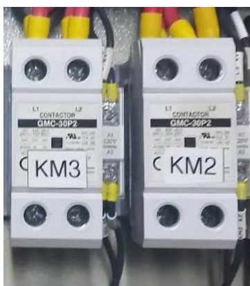
Figura 183 Contactor Metasol 2P, 30 A, 220 V
