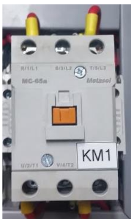
Figura 182 Contactor Metasol 65 A, 220 V
