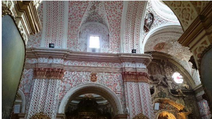
Figura 24: Interior Nave - Iglesia
