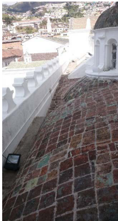
Figura 25: Tejuelos Exterior Nave Central
