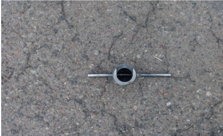
Figura 3.1 Extractor de pitch lock
