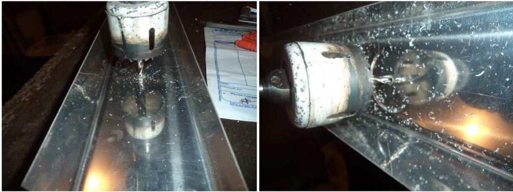
**Figura 3.18** Perforación floor beam
