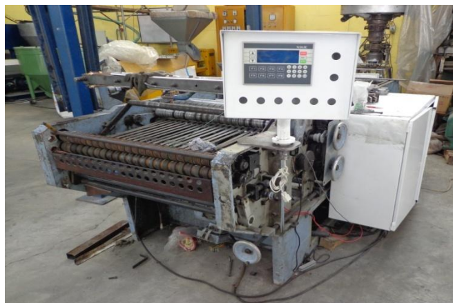
Figura2. 31: Tablero de Control
