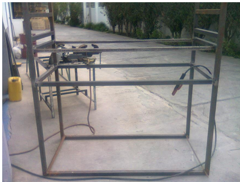
Figura 3. 3. Soldar bases faltantes
