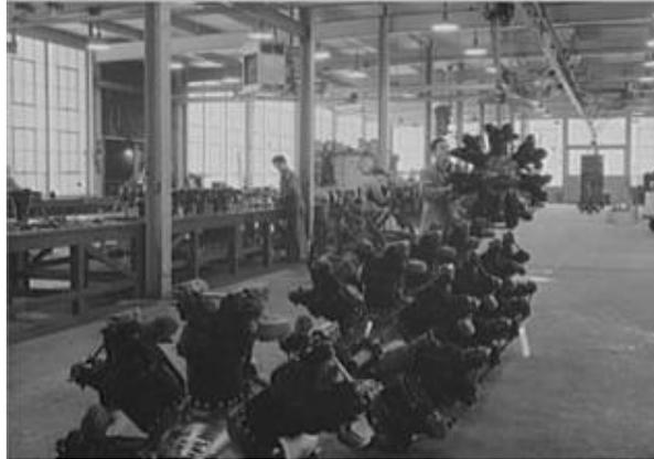
Nota. Motor A-70 radial, seven cylinder engine is introduced, (Continental, 1929).
