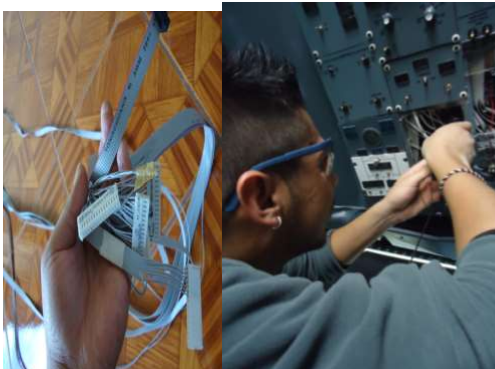
Figura 3.15 Implementation Del “CAUTION-ANNUNCIATOR WARNING LIGHT PANEL”
