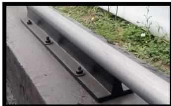
Fig. 18 ANCLAJE HACIA LA COLUMNA
