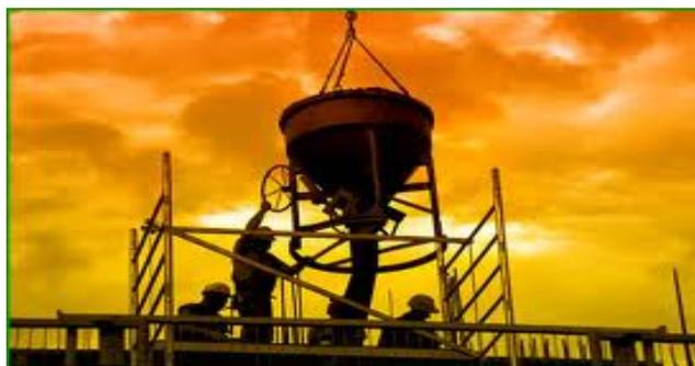
**FIGURA 23: EJEMPLO DE RESGUARDOS PARA IMPEDIR CAÍDAS**
