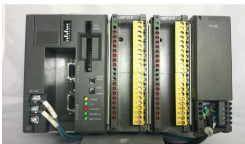
Figura 4 PLC Modicon 984-A120, Reactor MQ5
