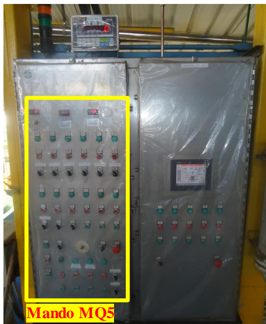
Figura 25 Tablero de control Reactor MQ6, mando MQ5
