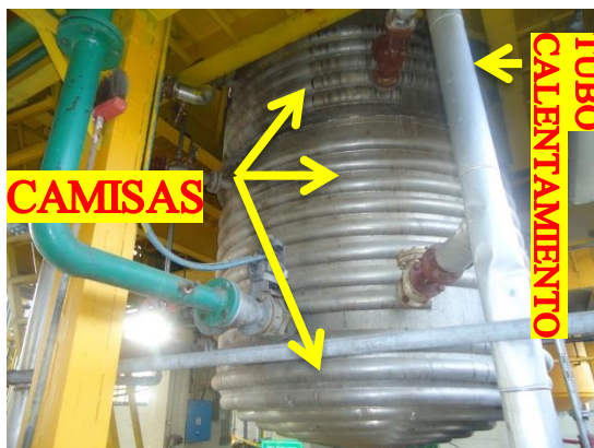
Figura 12 Camisas, Reactor MQ6
