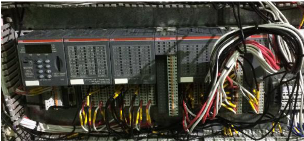
Figura 36 PLC ABB gama AC500 modelo PM573
