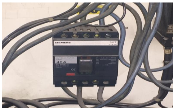
Figura 24 Breaker general máquina Van Dorn.
