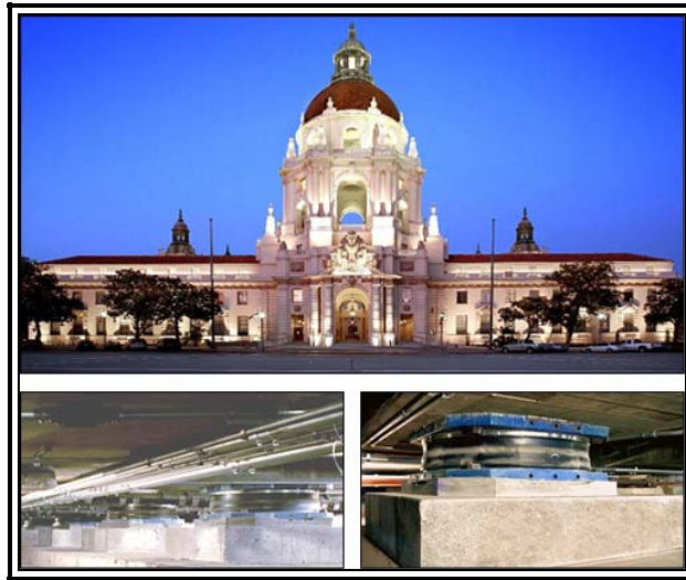
Figura 1.12: Pasadena City Hall, California
