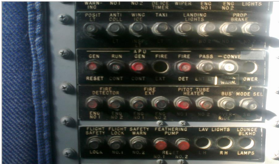
Figura 2.8: Panel de Circuits Breaker
