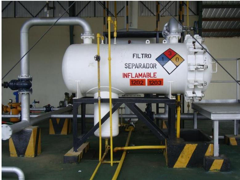
FIGURA 2.17 Micro separador Horizontal FRAM
