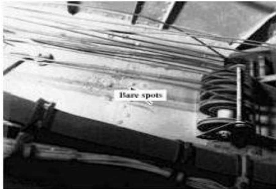
Figura 2.29: Cables de control
