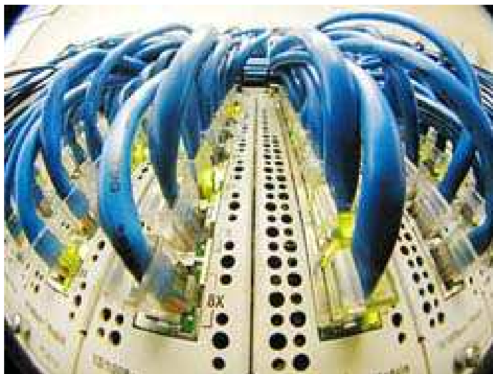
Fig.B-1 Patch Panel UTP
