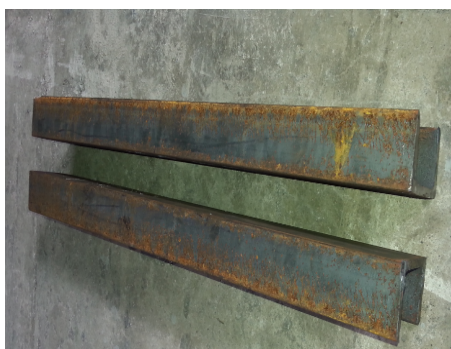
Figura 5.12: Viga principal (AC)
