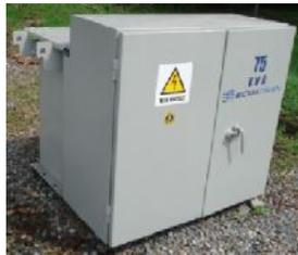
**Figura 4.32. Transformador Padmounted 75KVA**
