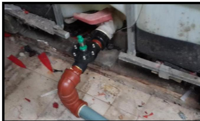
**Figura 75:** Acople electroválvula tanque 3
