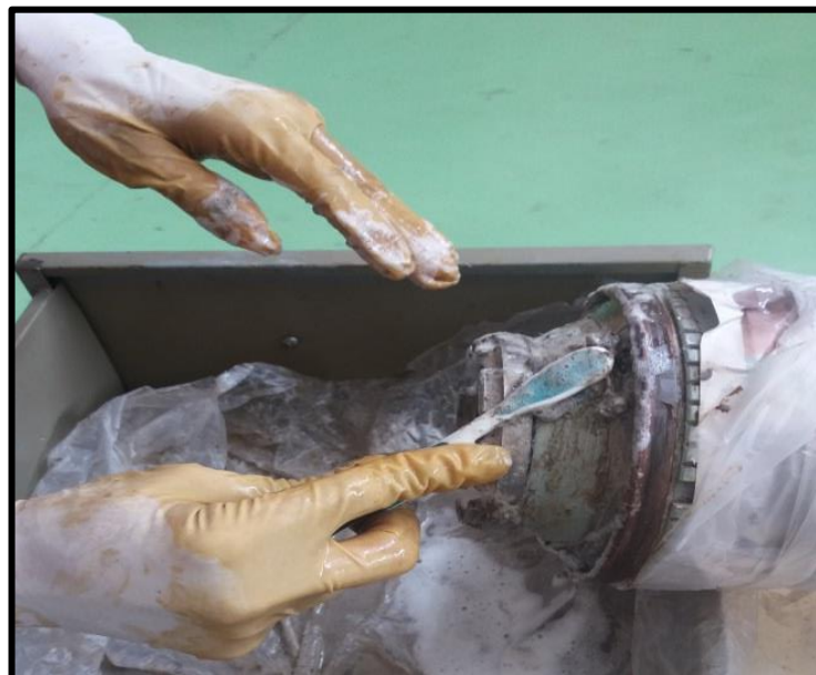
Figura 66: Blade and bushes assembly limpieza
