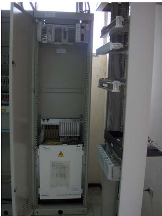
**Figura 1.35. Multiplexores Siemens TransXpress SMA-16**
