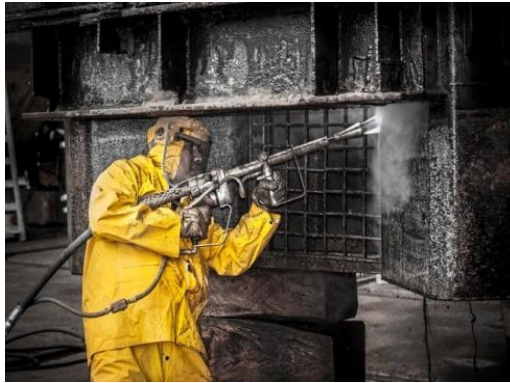
Figura 3.10 Waterblasting
