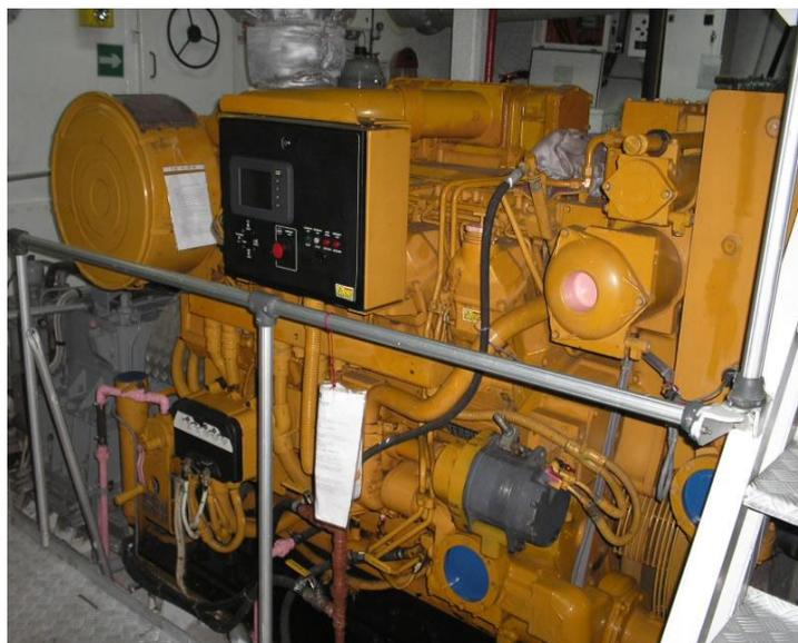
**Figura 1-5. Máquina principal Caterpillar 3508B.**
